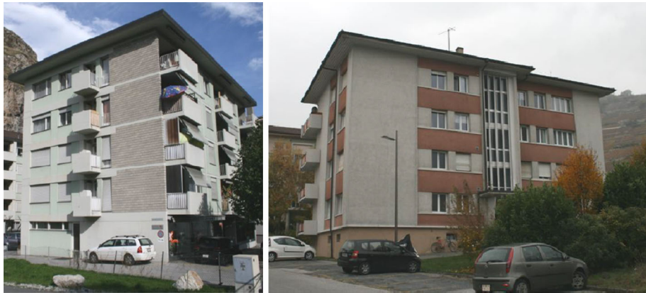
Fig. 2 Typical unreinforced masonry buildings in Switzerland
